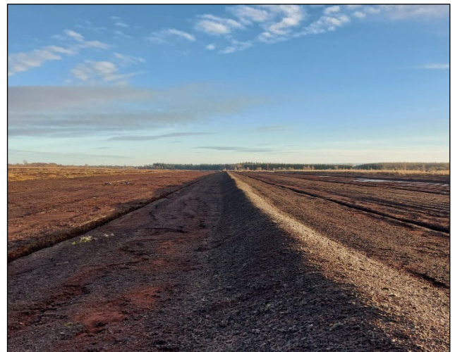
Plate 3-4 Stockpile at Derrynagun Bog.
