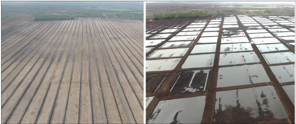
Example of pre and post rehabilitation showing significant rewetting (image left taken September 2021 and image right taken March 2023).
