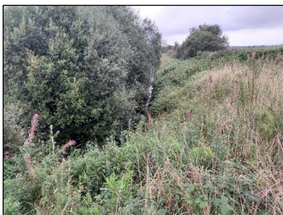
Example of large trench drains that run north-south through the site.
