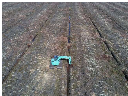
Figure 3.5. Northern-eastern section (2020). Drain-blocking and bog restoration
