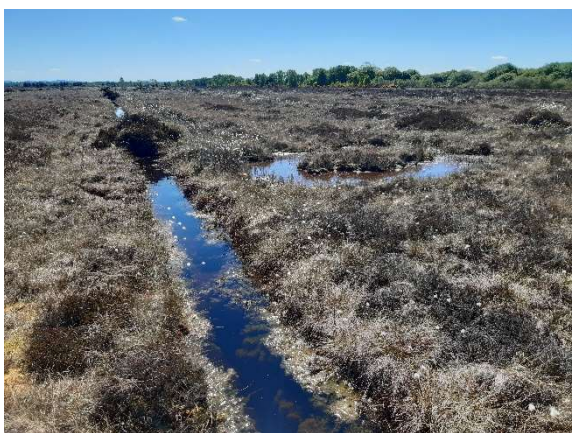
Figure 3.6. Northern-eastern section (2020). Drain-blocking and bog restoration
