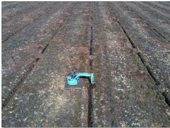
Image 3.5. Northern-eastern section (2020). Drain-blocking and bog restoration
