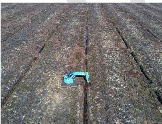
Figure 3.5. Northern-eastern section (2020). Drain-blocking and bog restoration
