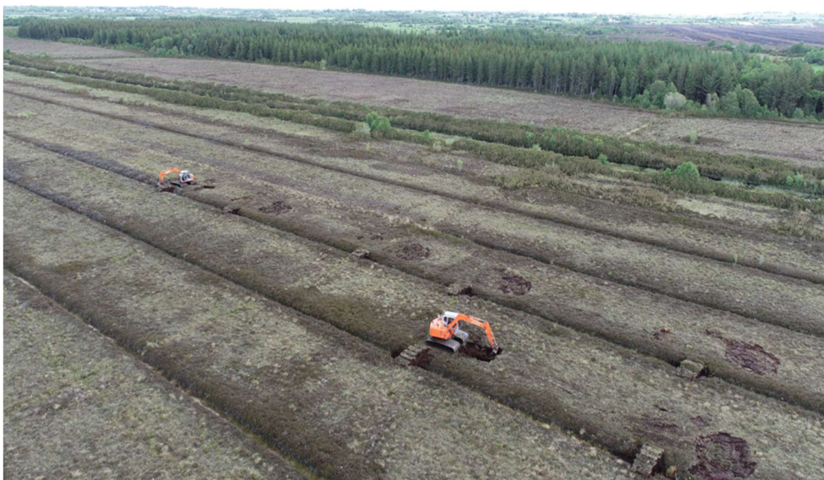
Figure 2: Drain blocking being carried out at Kellysgrove
