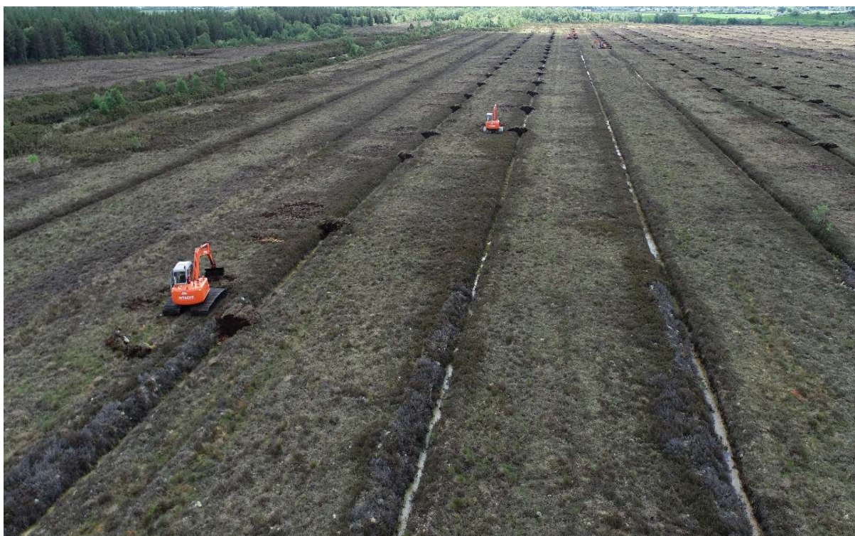
Figure 1: Drain blocking being carried out at Kellysgrove
