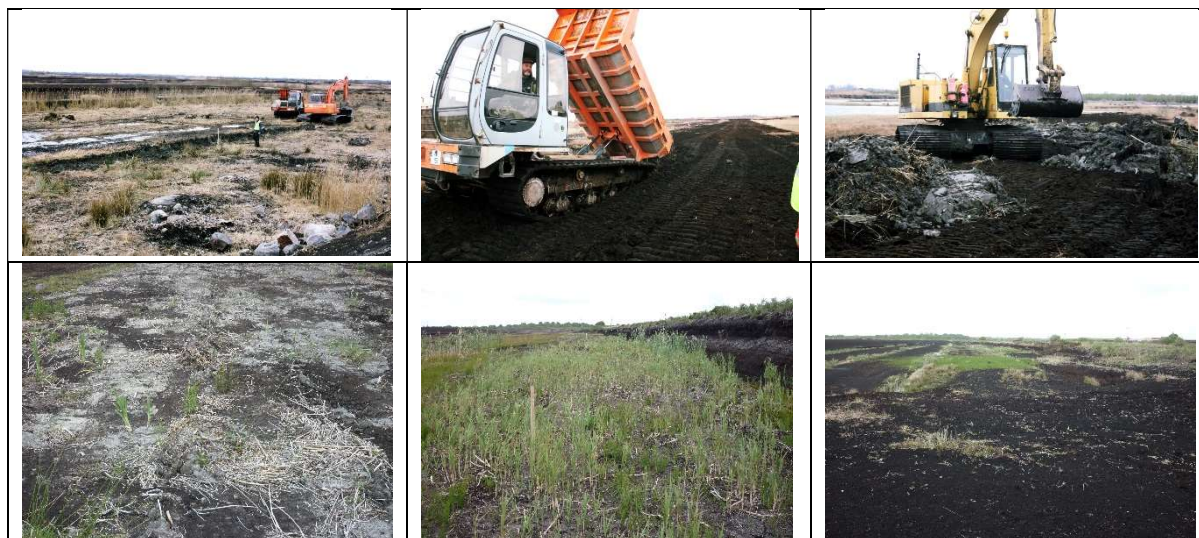
Figure 10.3. Blackwater bog. Reedbed creation trial spring 2010. The top pictures demonstrate the machinery used. The bottom pictures show the growth of the Reeds during the following summer.
