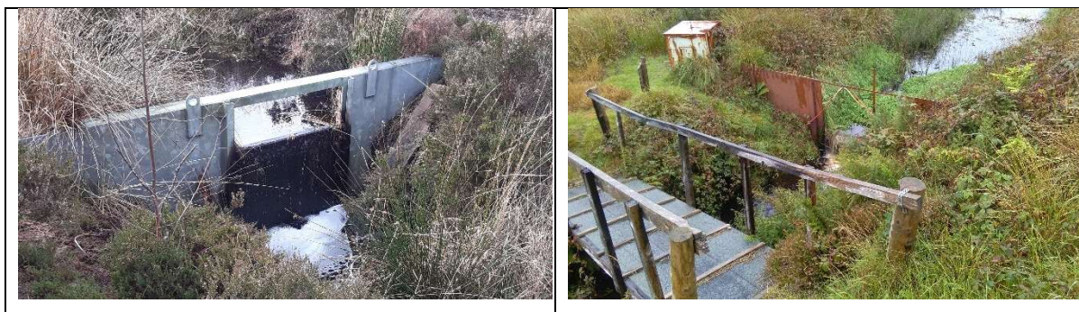
Figure B4.1. Types of controlled weir outfalls: Sluggan Moss (Bulrush) (left) and Srahmore (Bord na Móna) (right) with two different designs of drop board sluices.
