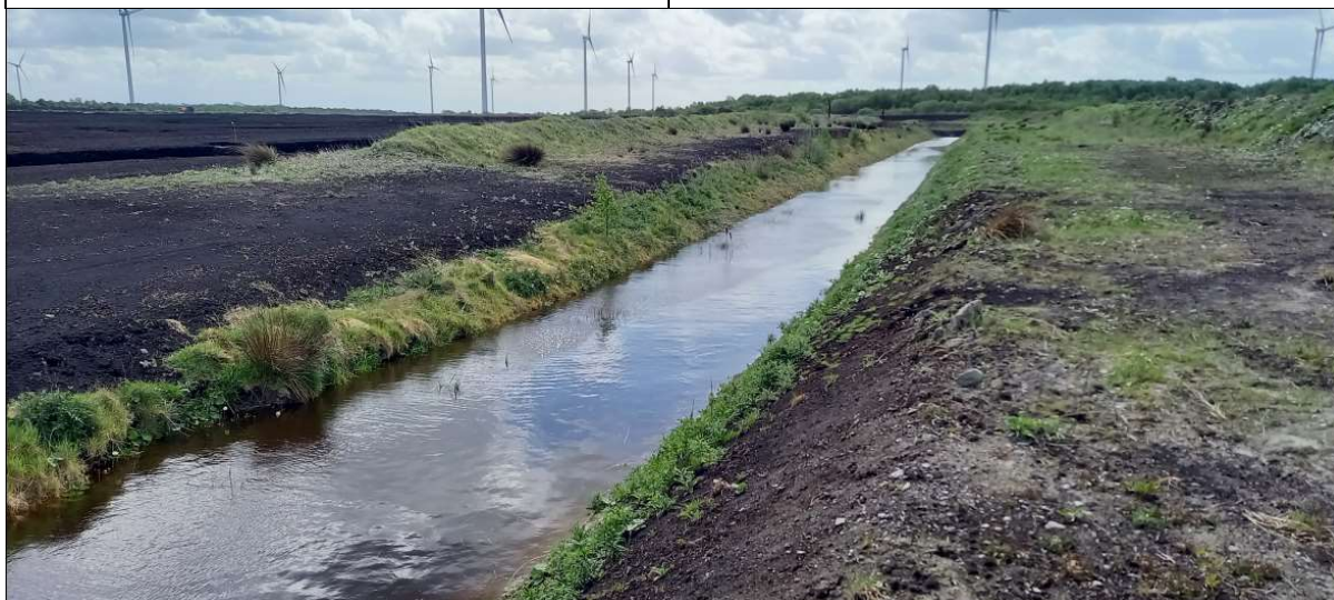
Figure 7.21. View of raised water level upstream of modified outfall.
