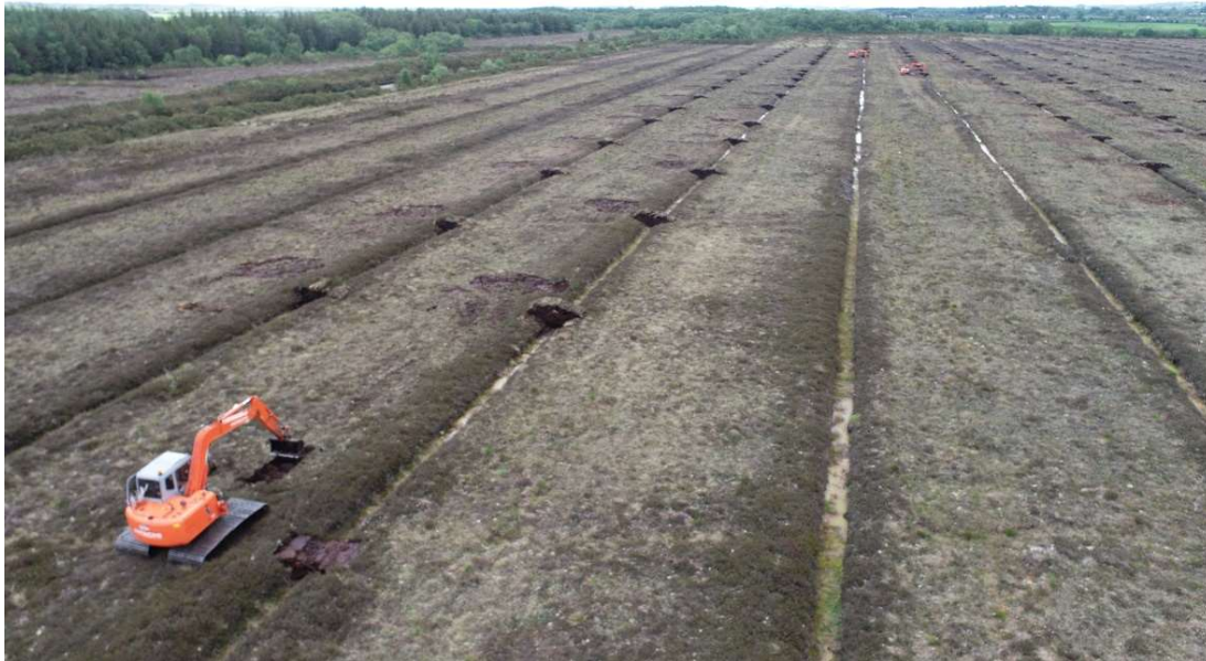
Figure 7.1. Kellysgrove Bog June 2021. Drain Blocks being formed.
