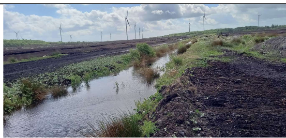
Figure 7.20. New water level in the outfall at Mountlucas.
