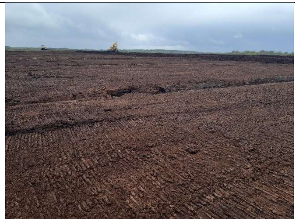
Figure 7.6. Levelled peat fields with camber removed.
