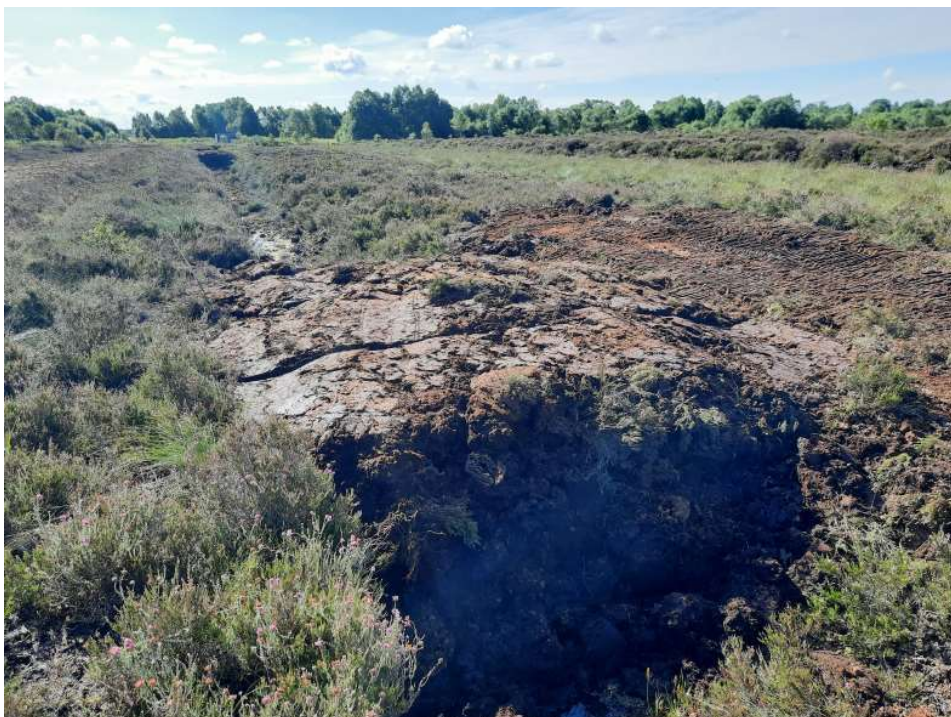
Figure 7.23. Trench drain at Glenlough Bog.
