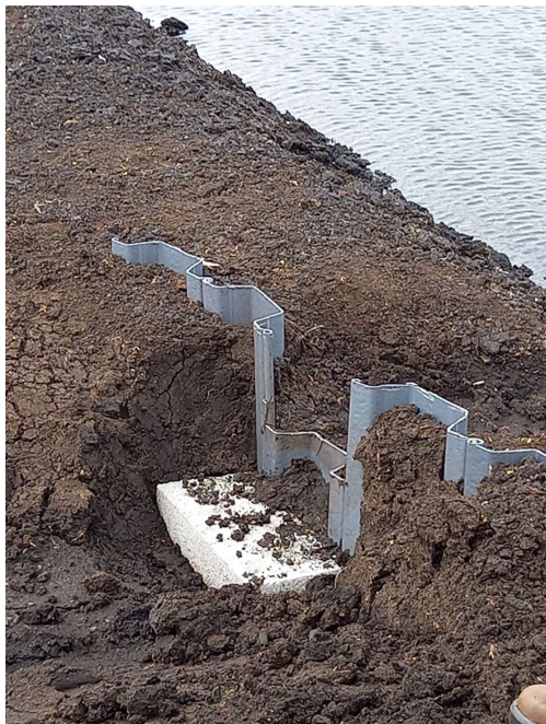
Figure 7.9. Sheet piles to regulate flow between cells – Belmont Bog.
