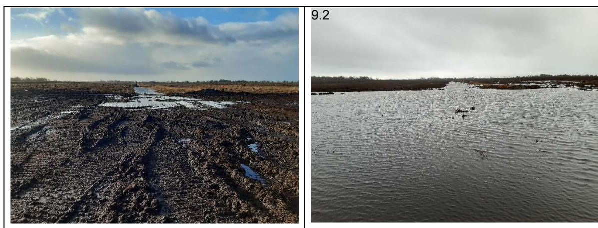
Figure B9.2. Line of trench drain at Derryhogan showing recent block in foreground (picture on left; Nov-19) and the same area c.10 weeks later (photo on right; Feb-20); note re-wetting on peatlands to either side of trench drain following installation of block.
