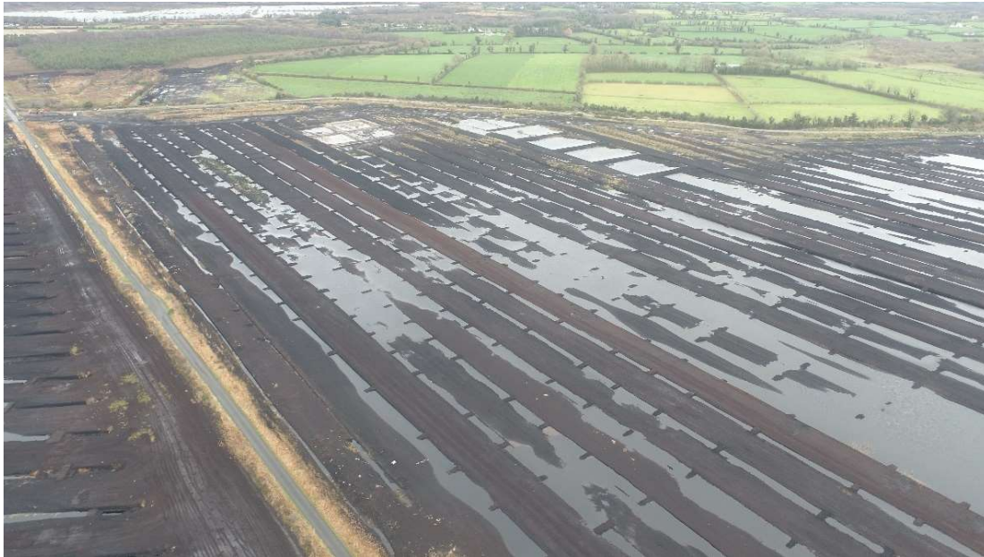
Figure 7.3. Drain blocks in Derrycolumb Bog.
