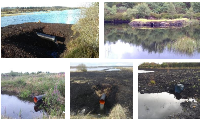
Figure 8: Examples of installed overflow pipes
