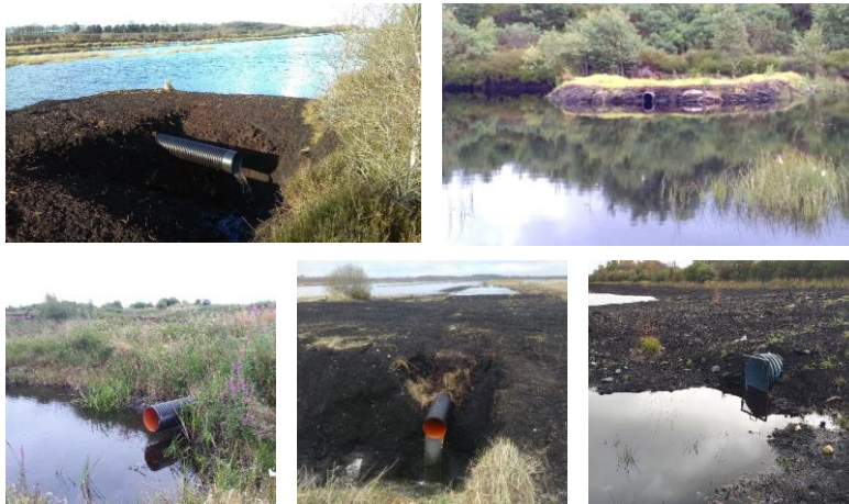
Plate 2-1: Examples of installed overflow pipes
