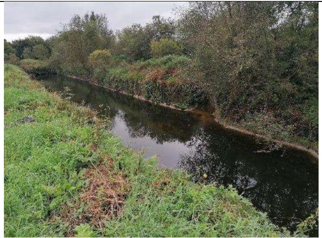
View of typical silt ponds in Bloomhill
