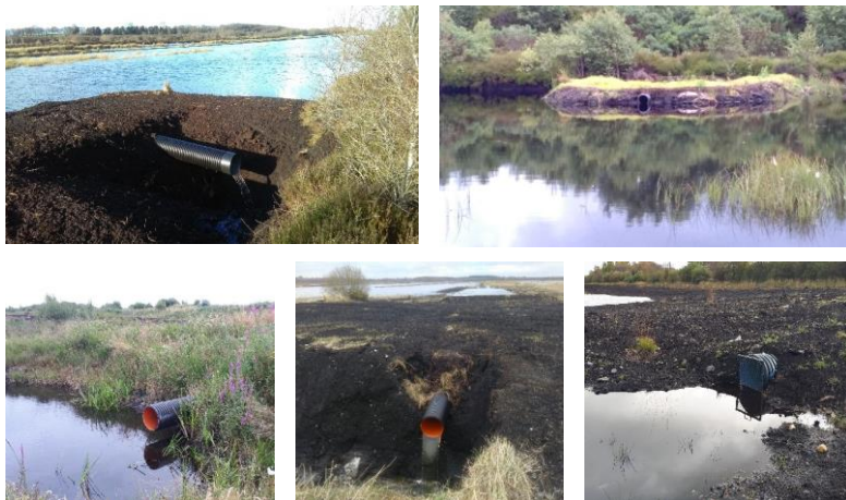
Figure 8: Examples of installed overflow pipes
