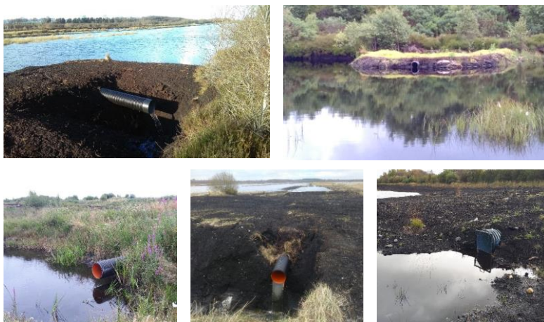
Figure 11: Examples of installed overflow pipes
