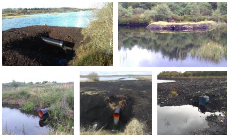
Plate 2-2: Examples of installed overflow pipes
