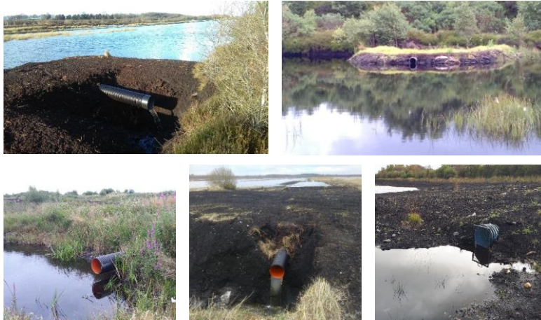
Plate 2-2: Examples of installed overflow pipes
