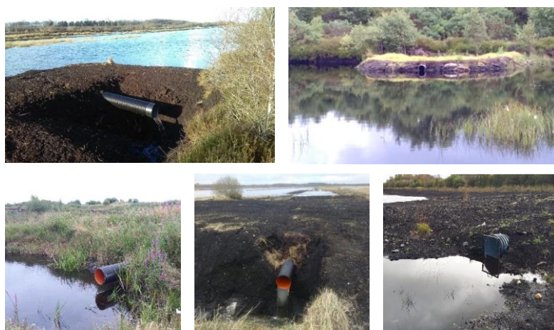
Figure 8: Examples of installed overflow pipes
