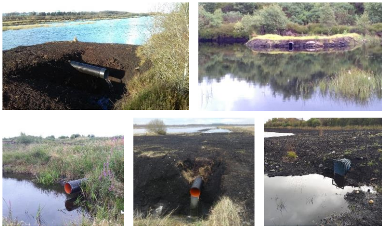
Figure 11: Examples of installed overflow pipes
