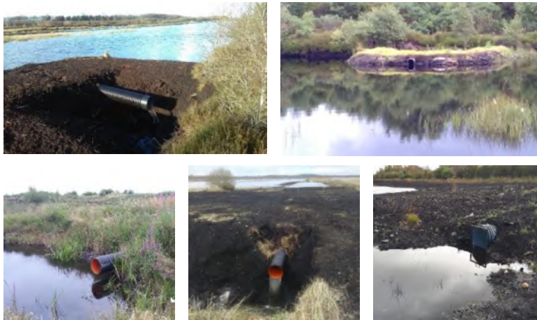
Plate 2-2: Examples of installed overflow pipes
