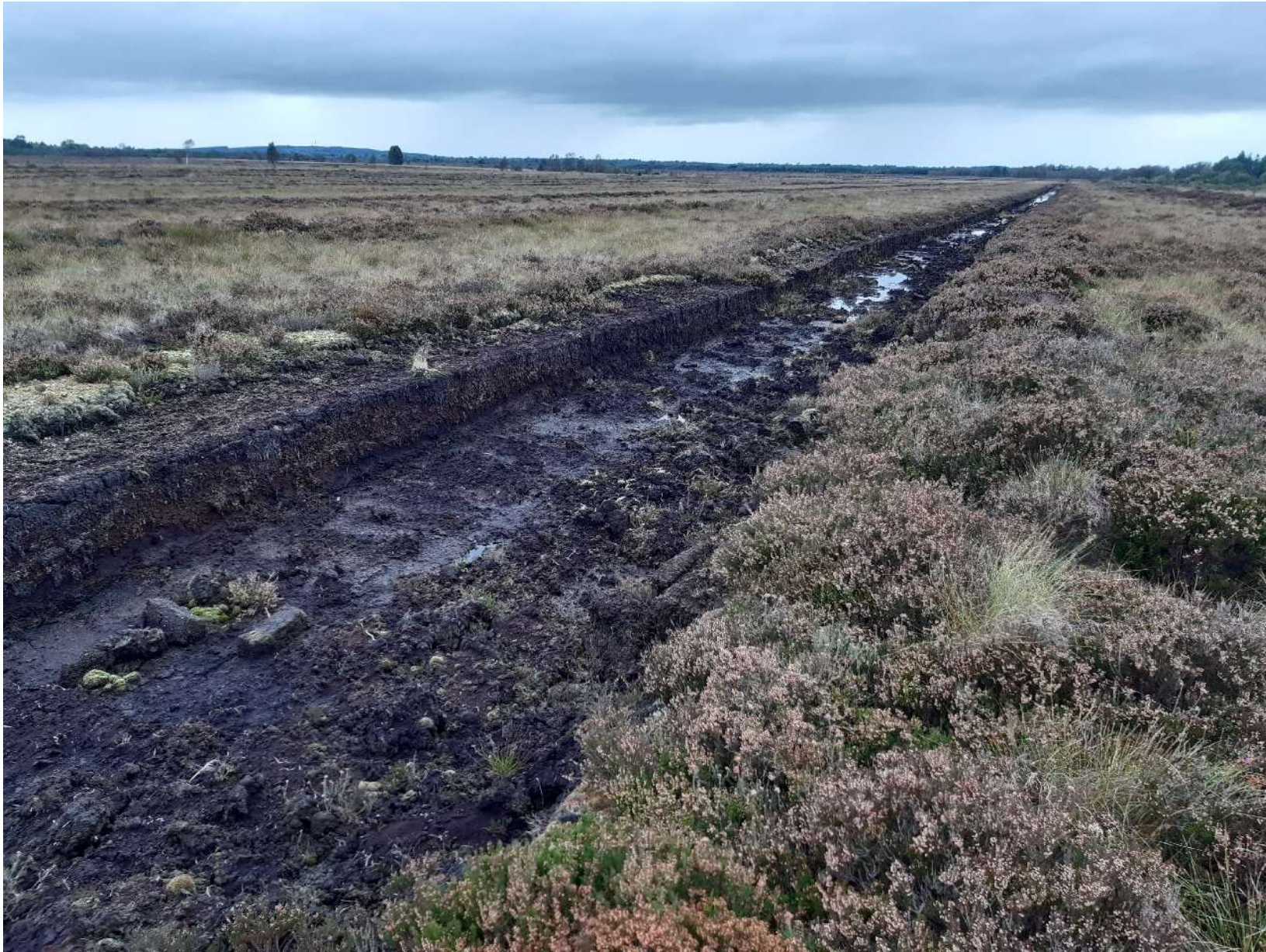
Figure 3.1. View of large trench drain present in Glenlough
