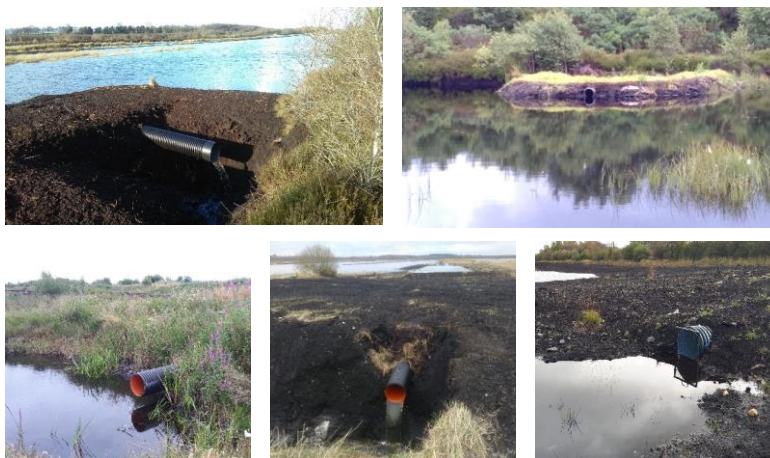
Plate 2-2 Examples of installed overflow pipes
