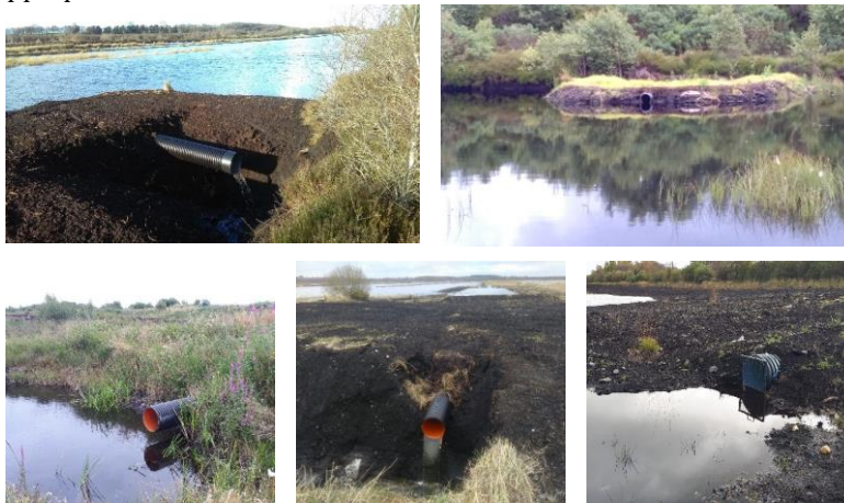
Plate 2-2 Examples of installed overflow pipes
