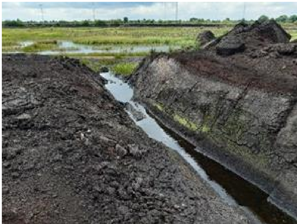
Figure 5.5.1.1 'V' Tap across a high field at Baunmore to control water levels
