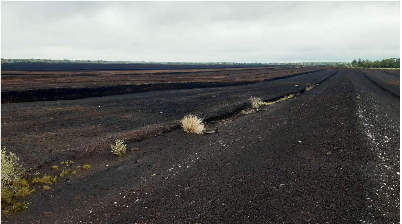
Figure 3.3. View of the typical milled peat surface with existing drainage across Clooniff Bog
