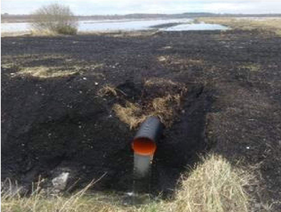
Figure 5.5.3.1 Raised water outlet at Cavemount
