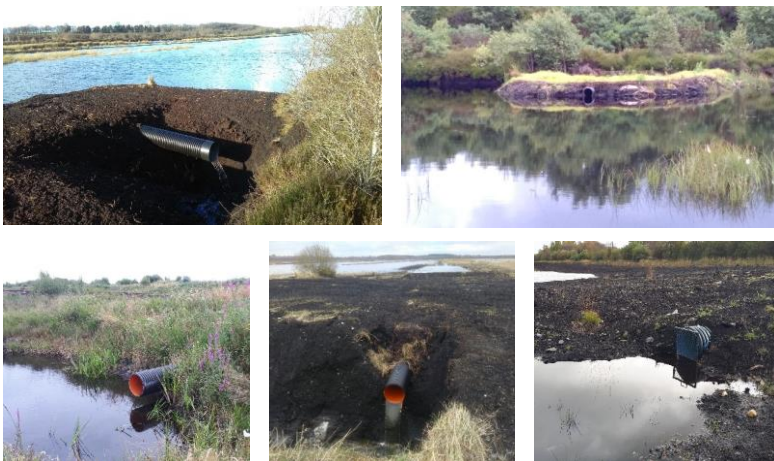
Figure 8: Examples of installed overflow pipes
