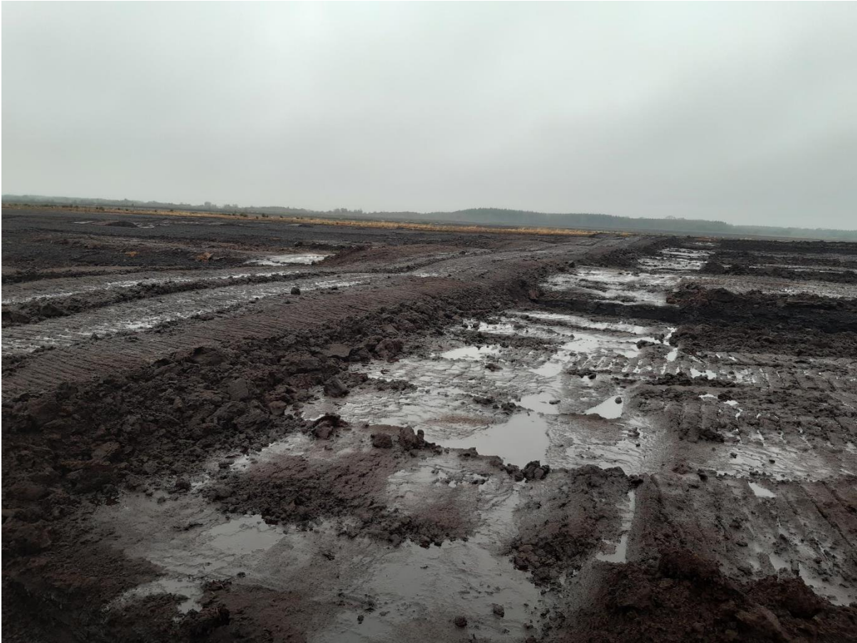
Figure 5.3.1 Peat Berm at Castlegar Bog
