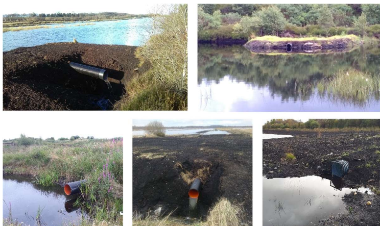
Figure 7: Examples of installed overflow pipes
