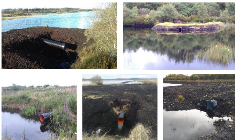
Plate 2-2: Examples of installed overflow pipes
