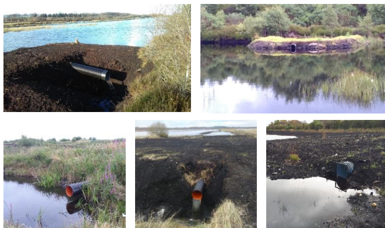
Figure 7: Examples of installed overflow pipes
