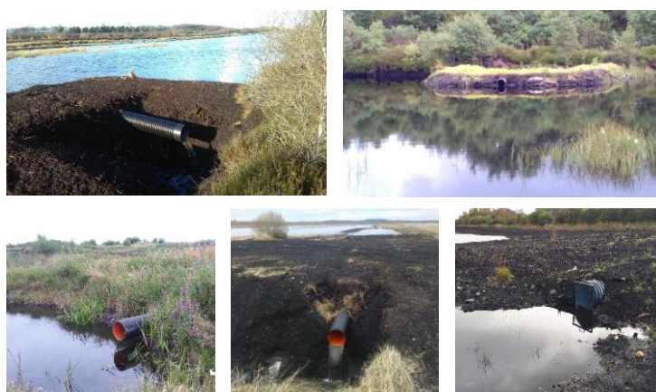
Plate 3: Examples of installed overflow pipes
