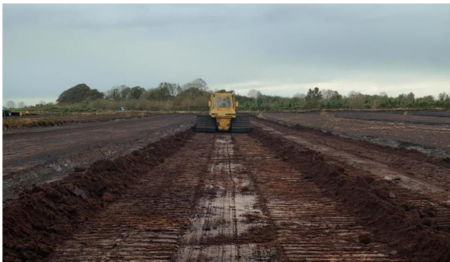
Figure 5.4.2 Field re-profiling using Bulldozer Only
