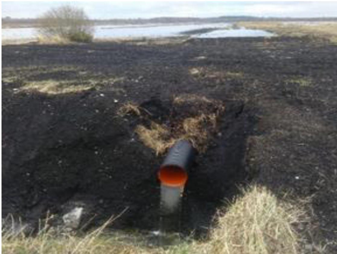
Figure 5.6.3.1 Raised water outlet at Cavemount
