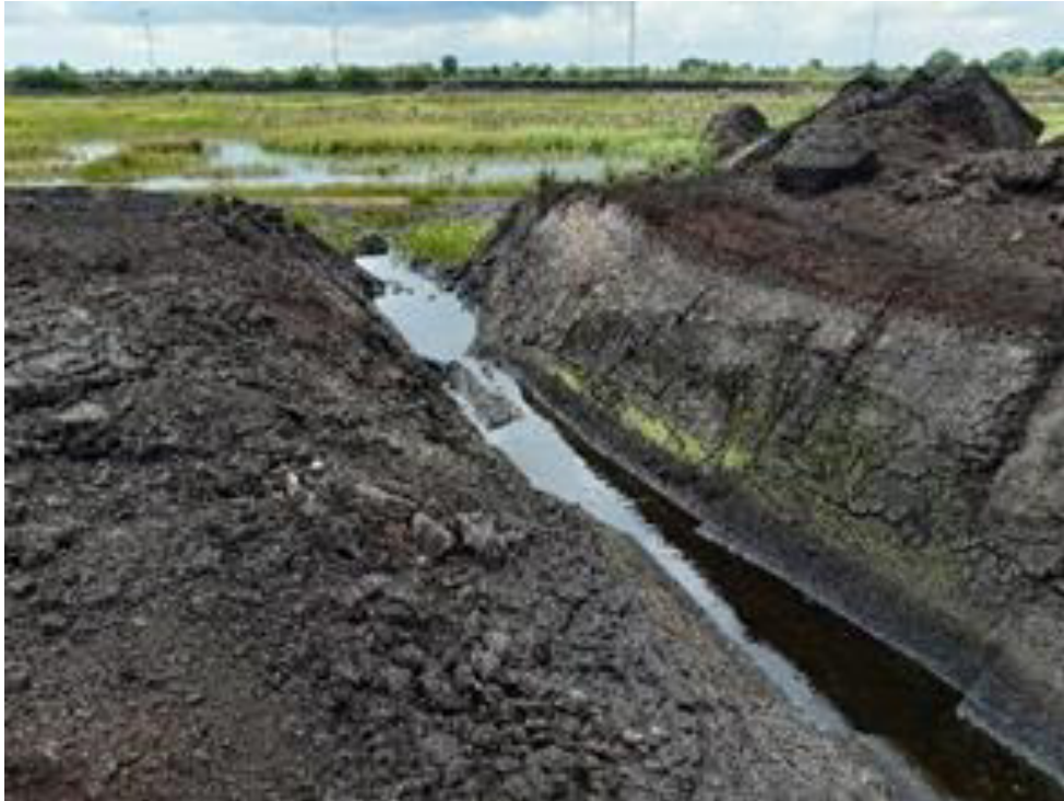
Figure 5.6.1.1 'V' Tap across a high field at Baunmore to control water levels
